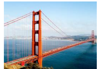
GOLDEN GATE BRIDGE
